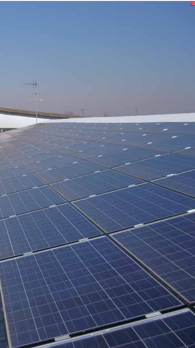
13. GMN Stand alone PV array at Nembrala (Indonesia) 21 kWp (Sunnyspain®Hybrid)
