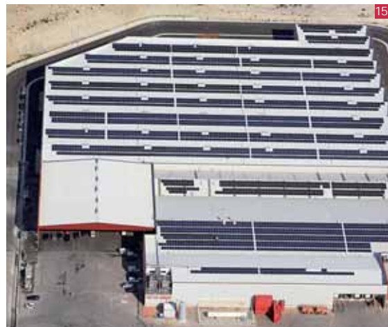
15. GRUPOTEC SOLAR PV array on an industrial roof at Molina de Segura (Spain) 990 kWp (9 Sunnyspain®Sun 100)
