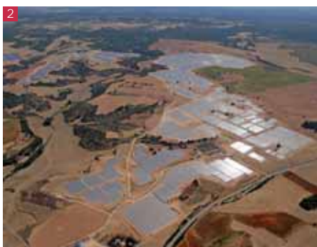
2. NOBESOL PV array at Olmedilla de Alarcón (Spain) 60 MWp (453 Sunnyspain®Sun 100 )
