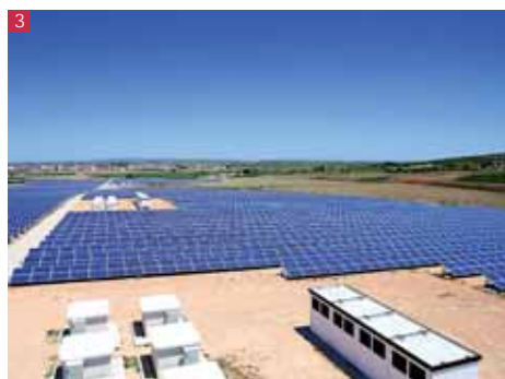
3. FV3 PV array at Pocico Salao (Spain) 5.16 MWp (16 Sunnyspain®Sun 25 , 33 Sunnyspain®Sun 100 )
