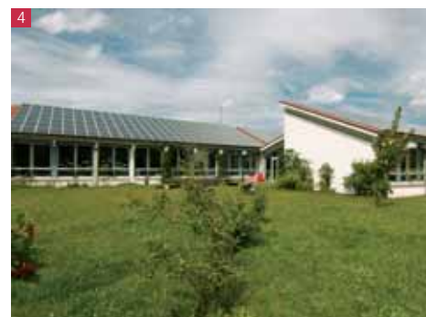
4. SAILER GmbH PV array at Asch (Germany) 82.95 kWp (14 Sunnyspain®Sun 4.6TL )
